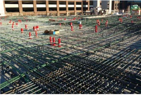
The result is that the tendons, like rubber bands, want to return to their original length but are prevented from doing so by the permanent anchorages. The permanently stressed state of the tendons results in a compressive force acting on the structural concrete.
