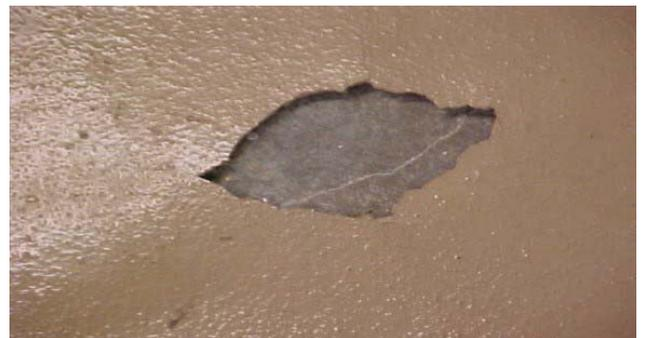
*Alkalinity is the most destructive water problem. Tests of adhesives commonly used for bonding floor finish to concrete slabs indicate that they lose a large portion of their dry bond strength when the concrete becomes damp. This is possibly due to chemical degradation of the adhesive at the junction of the adhesive and the concrete, and may be caused by a reaction, in the presence of water, between alkali in the cement and the resin in the adhesive.*
