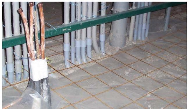
*Vapor retarders used under concrete slabs on ground restrict the flow of moisture vapor from the sub-grade into and through the slab.*
