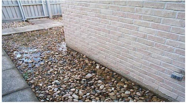
*Poor exterior drainage allows water accumulation at the base of an exterior wall and infiltration of water under the interior floor slab that can saturate floor coverings around the interior perimeter of the building.*
