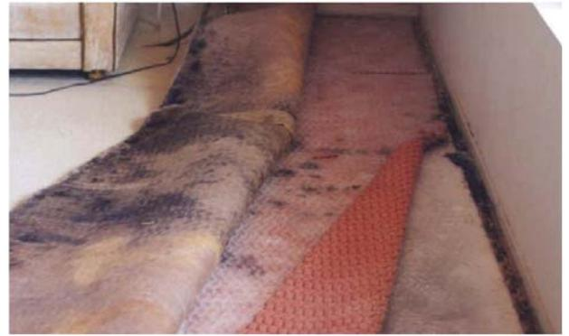
*Microbial Growth – Excessive moisture trapped under floor finishes can create conditions for mold and mildew to grow.*
