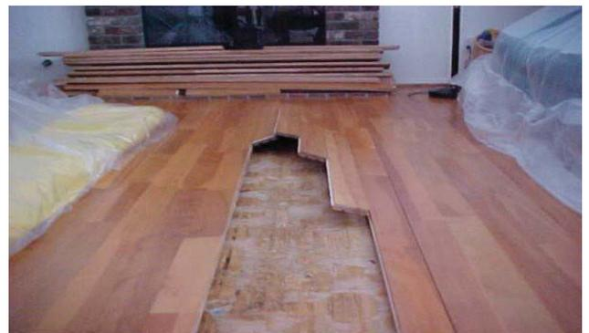
*Wood Expansion – Wood flooring glued directly to a damp concrete floor slab absorbed moisture from the slab, expanded, and buckled.*
