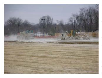
Cement, lime, and LDK are the most commonly used soil stabilization materials. When added in sufficient quantities, lime or LKD causes a chemical reaction with the clay base soils, the end result of which is a "glue" (pozzolan) that binds the soil particles together.
