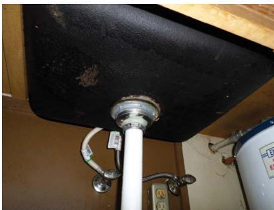
*Lesser known asbestos-containing building materials such as sink coatings and window glazing are now more closely scrutinized by regulators.*
